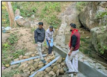
2 Jan 2026 | Kamrup: Team plot inspection visit for Diversion-Based Irrigation (DBI) intervention at Goleya village, Kulsi, Kamrup.
